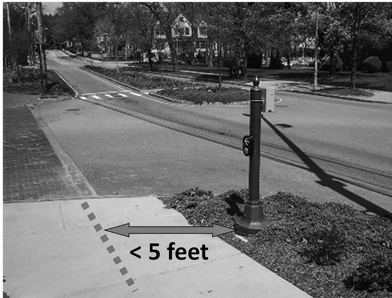
Figure 2. Pushbutton Location Within 5 Feet of Crosswalk
