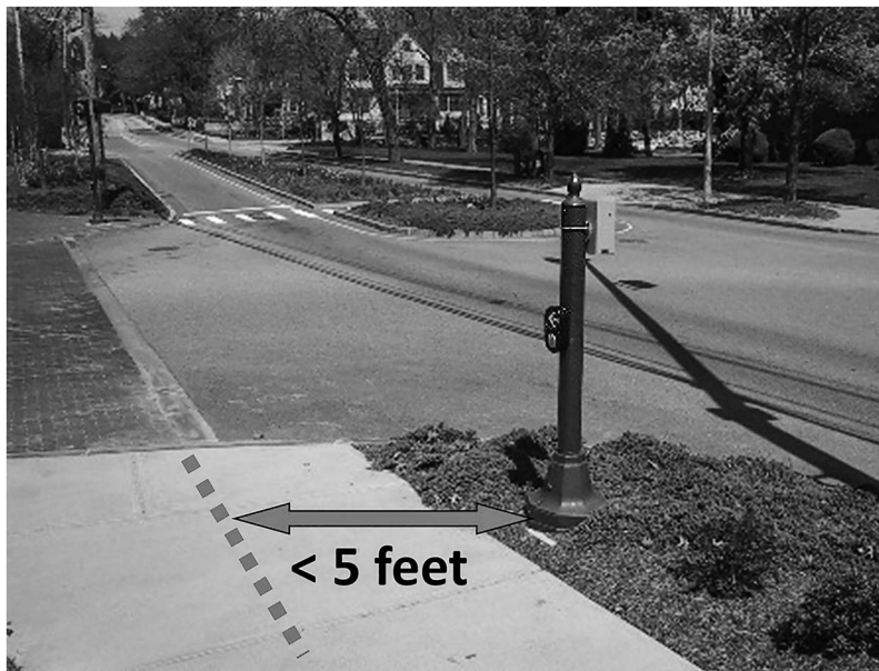
Figure 2. Pushbutton Location Within 5 Feet of Crosswalk
